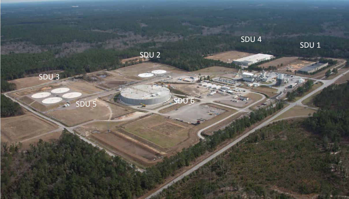
Fig. 1. Saltstone Production Facility, showing the Saltstone Disposal Units (SDUs).
