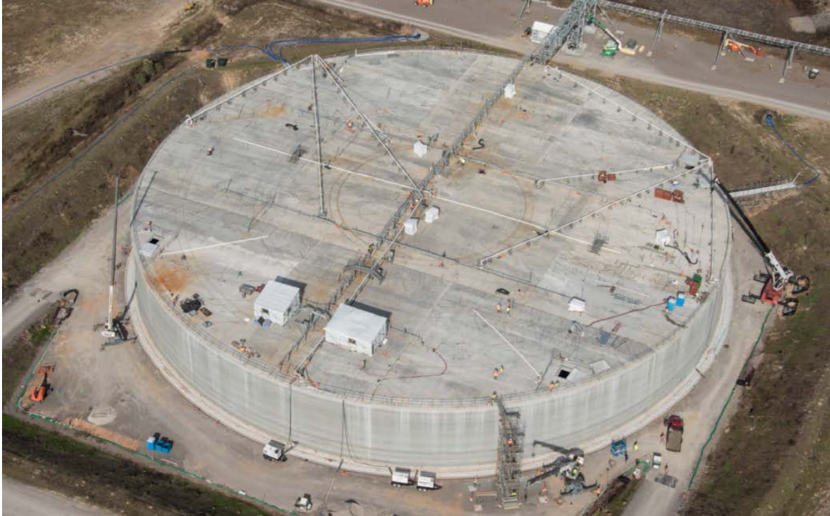
Fig. 3. SDU-6 near completion.
