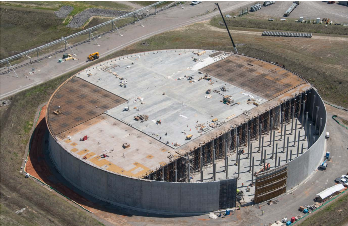
Fig. 2. SDU-6 during construction.
